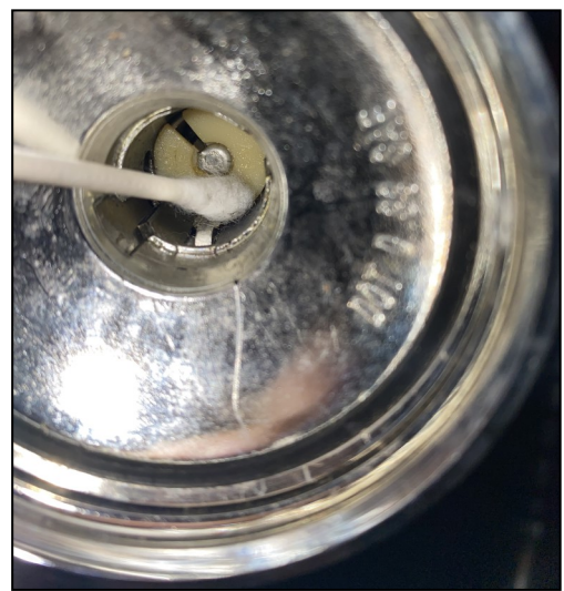
Using a NON CONDUCTIVE item, make sure the socket spring is moving up and down freely.
